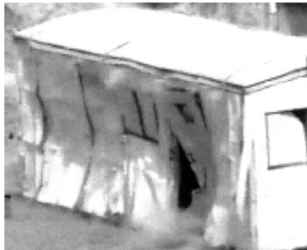
Figure 5.8. High speed photograph of building being deformed by pressure from a bomb explosion
