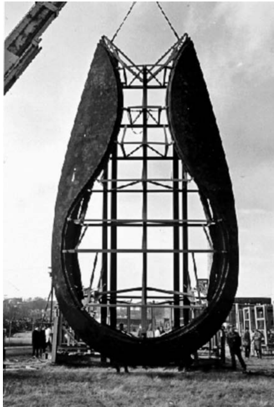
Figure 5.1. Sonar rubber bow dome
